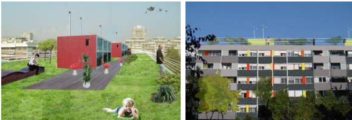
Fig. 14. Green roof; wind turbines and PV panel integration in the façade
