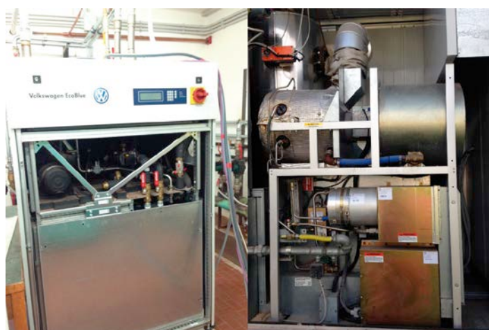
Figura 6 – CHP Volkswagen e MGT Capstone
