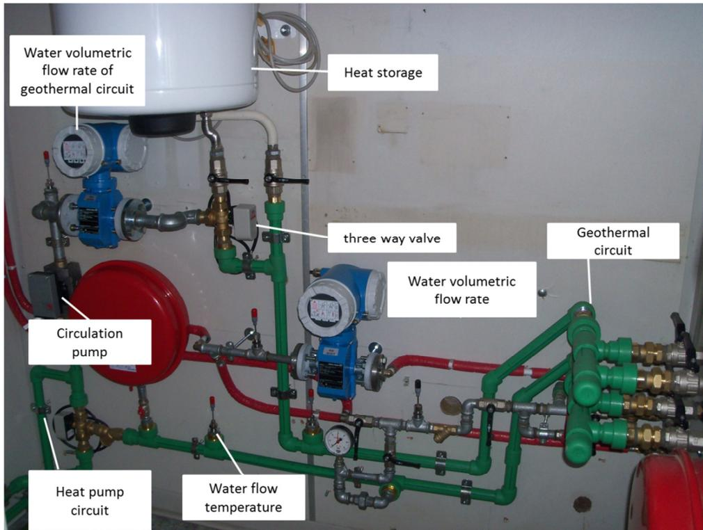
Fig. 2 - Plant hydraulic scheme
